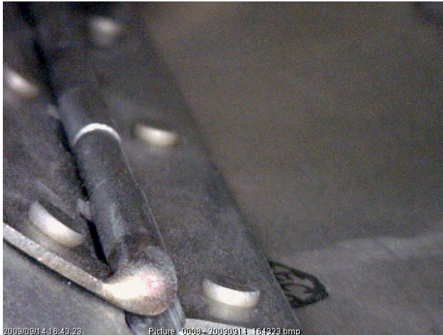
Welded hinge pin retention.
